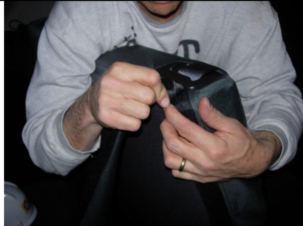
Step 15. Driver Top/DT: Tuck the fabric under the plastic for the seat belt, then connect the Velcro™ at the top.
