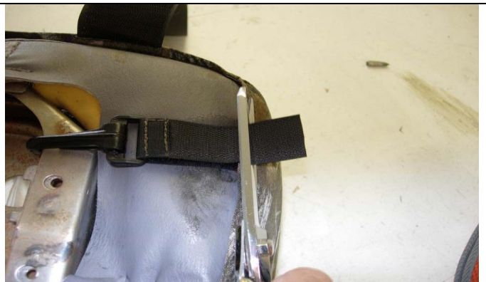
Step 12. Bottom: Carefully trim the excess length of Velcro™ with a scissor.
